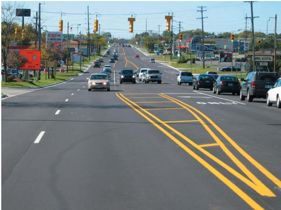
**Miller Road was completely reconstructed with 10 inches of full-depth asphalt.**
