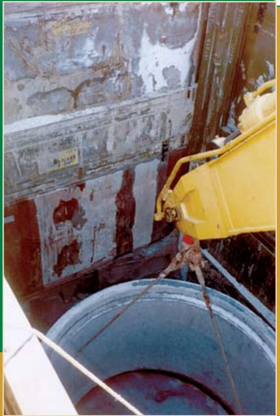
the triple rail configuration keeps side panels to a manageable, minimal weight. This helps in installation and removal. It's certainly easier than installing and
