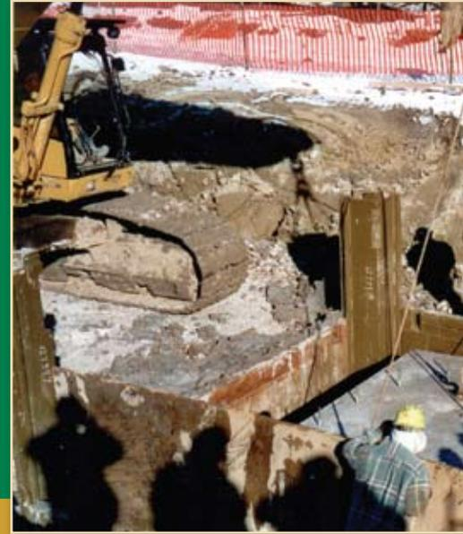
*Careful and skilled operation is required to lower the only 14 in. of clearance on the short side!*
